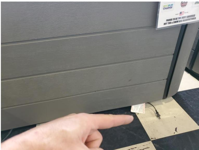
Reinstall the skirting on the spa and let the cord hang out the corner of the skirting. Plug in and heat for at least 24 hours before filling. We recommend you leave the heater in once full of water and running (unplugged) and tuck the cord up into the corner should you ever need to use it in your spa in the future.
